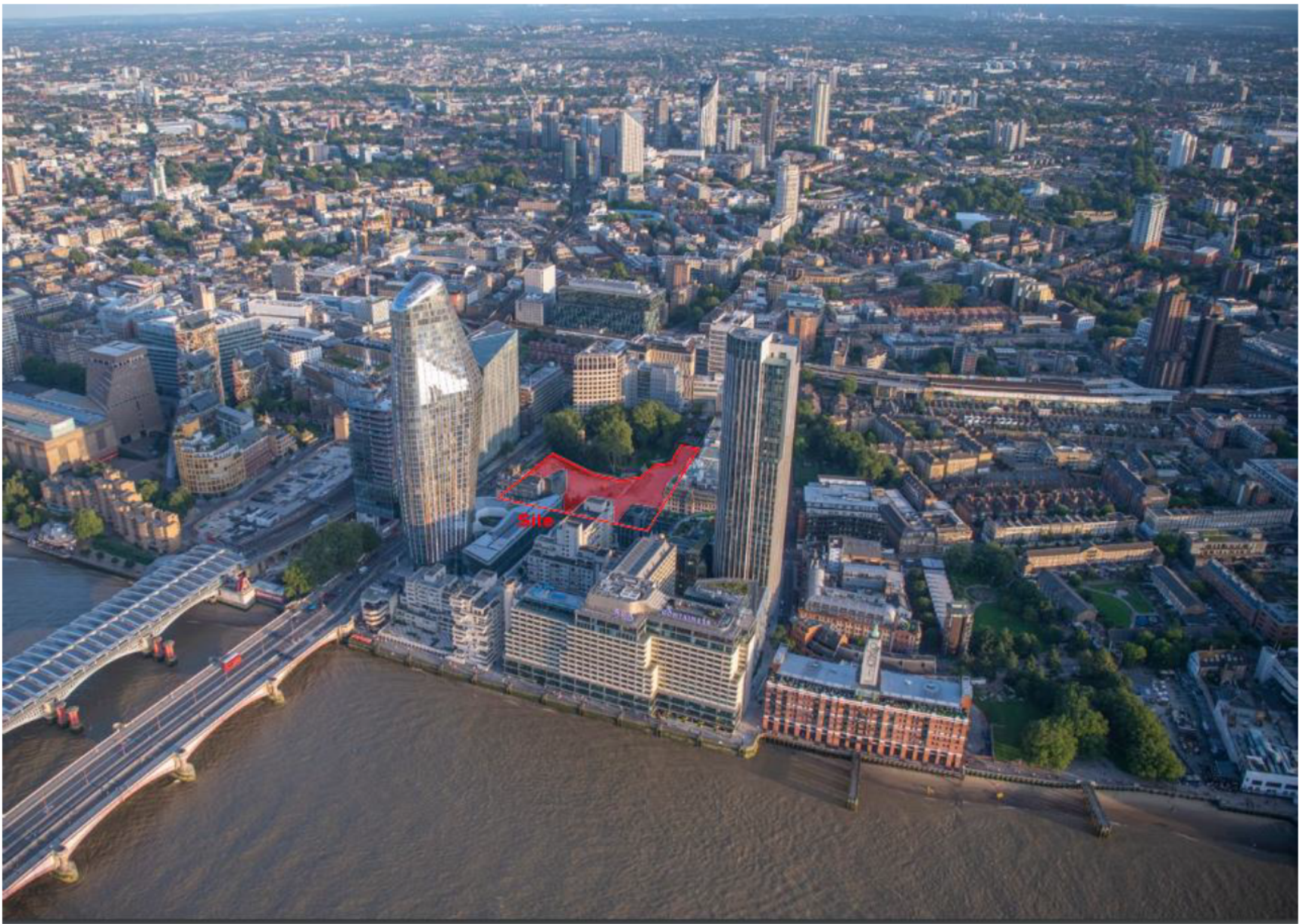
Aerial view looking south
